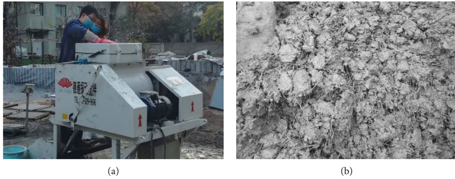
FIGURE 1: Mixing process of steel fiber concrete by vibratory mixing.
