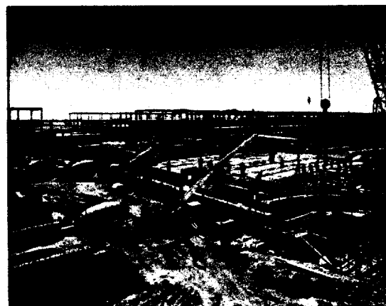
Figure 10: Casting a large volume (1100 m 3 ) suspended slab, using four lorry-mounted boom pumps which are fed directly by discharge from ready-mixed concrete trucks. (Photograph by courtesy of John Laing Construction Limited).
