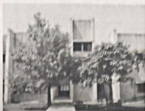
Fig. 1 A two storied building constructed using fly ash based concrete in 1973 at SERC, Chennai
