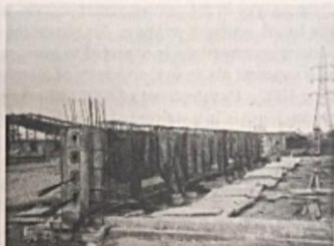
Fig. 9 A view of prestressed concrete fly over bridge girder cast using GGBS based HPC.
