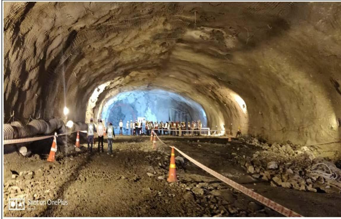
Photograph After Primary lining
