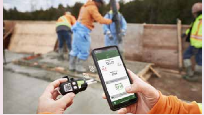
(fig-5 Monitoring of concrete temperature)
