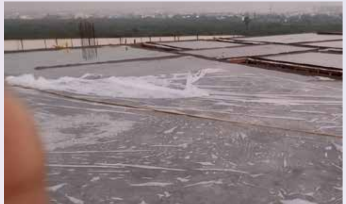
(fig - 1 Spreading of plastic sheet on concrete surface immediately after finishing)
