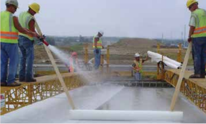
(fig - 3 Covering concrete surface with kraft paper)
