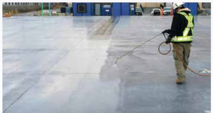
(fig-2 Application of curing compound after finishing)
