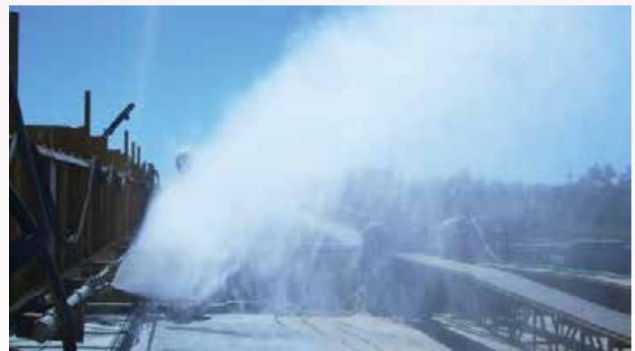
(fig-6 Method of steam curing)
