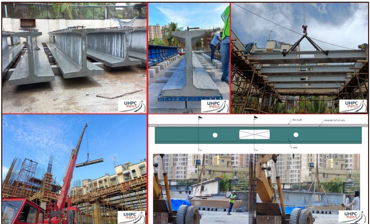
GCC Clubhouse – UHPC Beams, Mira Road, Mumbai
