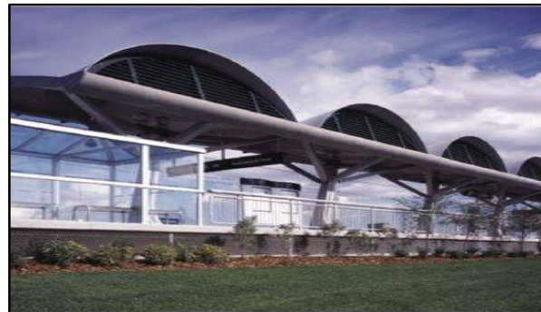
Shawnessy LRT Station, Roof in Canada
