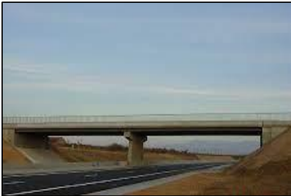
Bourges-les-Valence Road Bridge in France
