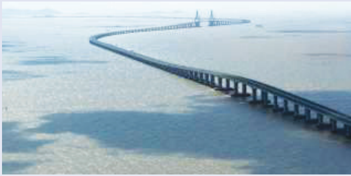
HPC - Hangzhou Bay Bridge, China - 36 km long bridge with predicted service life more than 100 years (High durability) (Constructed in 2007)
