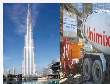
HPC – World record vertical pumping of 601 m with single pump (High workability)
