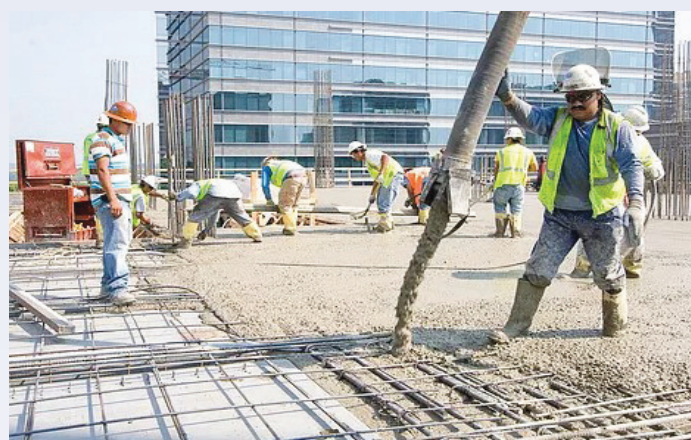
Pumpable Concrete Placement at Site
