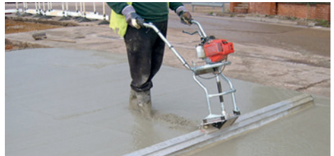
Figure 13. Petrol powered single beam screed
