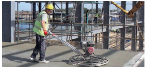
Figure 14. Power trowelling for a hard wearing finish.
